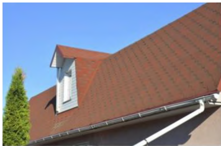
STRUCTURAL COMPONENTS (FLOORS, WALLS, ROOFS, FOUNDATIONS, ETC.).
